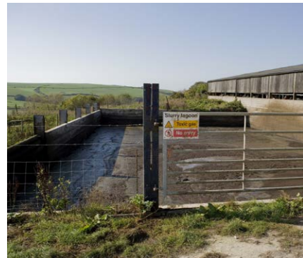
Leakage from slurry lagoons
