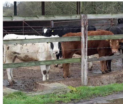
Drain connecting dirty farm yard to ditch
